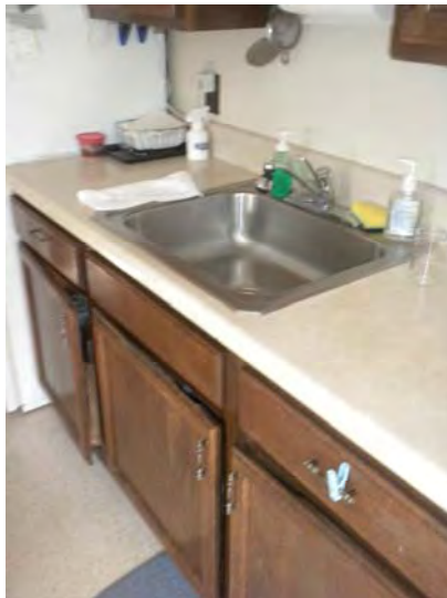
Plywood cabinetry and laminated particleboard countertops
